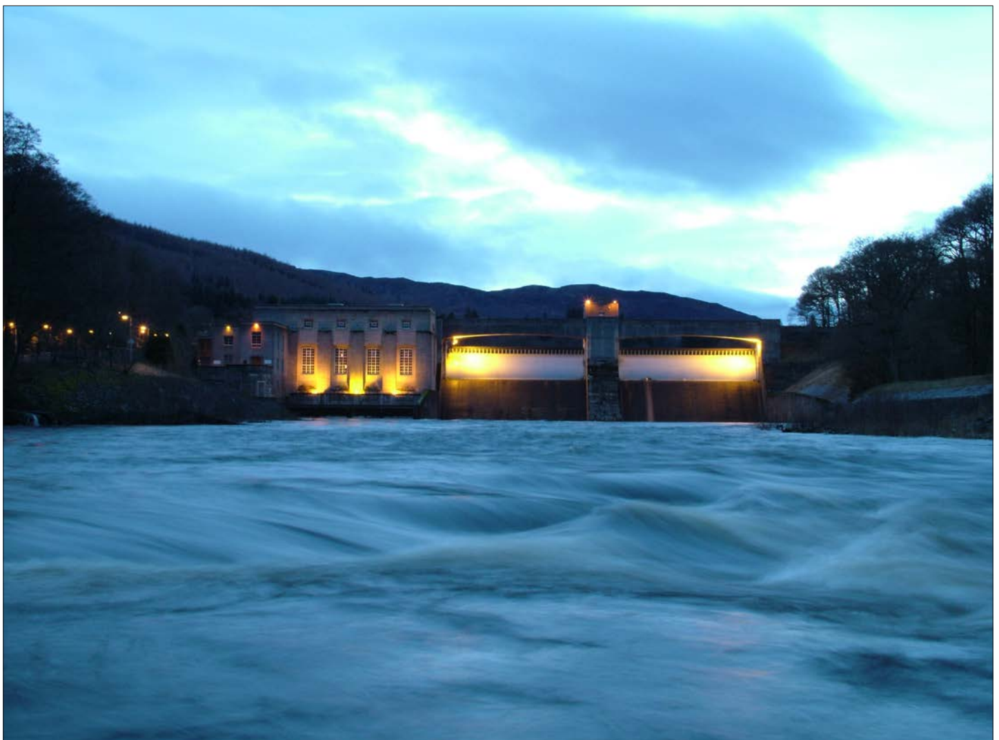
Above: SSE's Pitlochry hydro-electric power station
