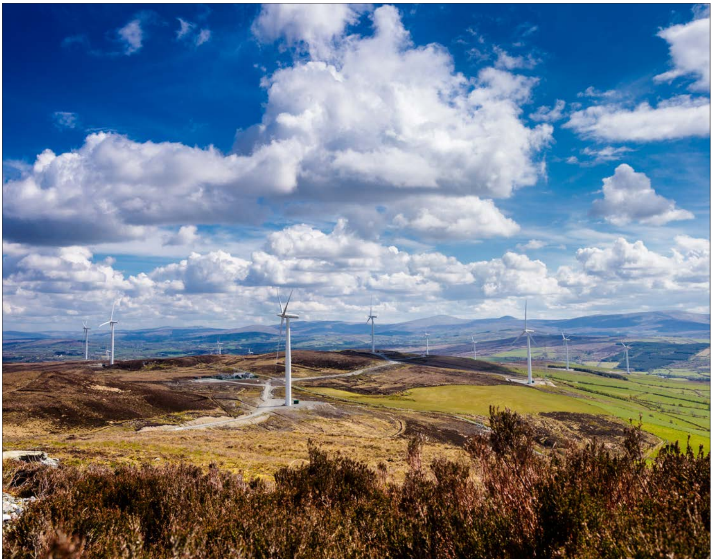
Above: SSE's Slieve Kirk Wind Park, the largest in Northern Ireland
