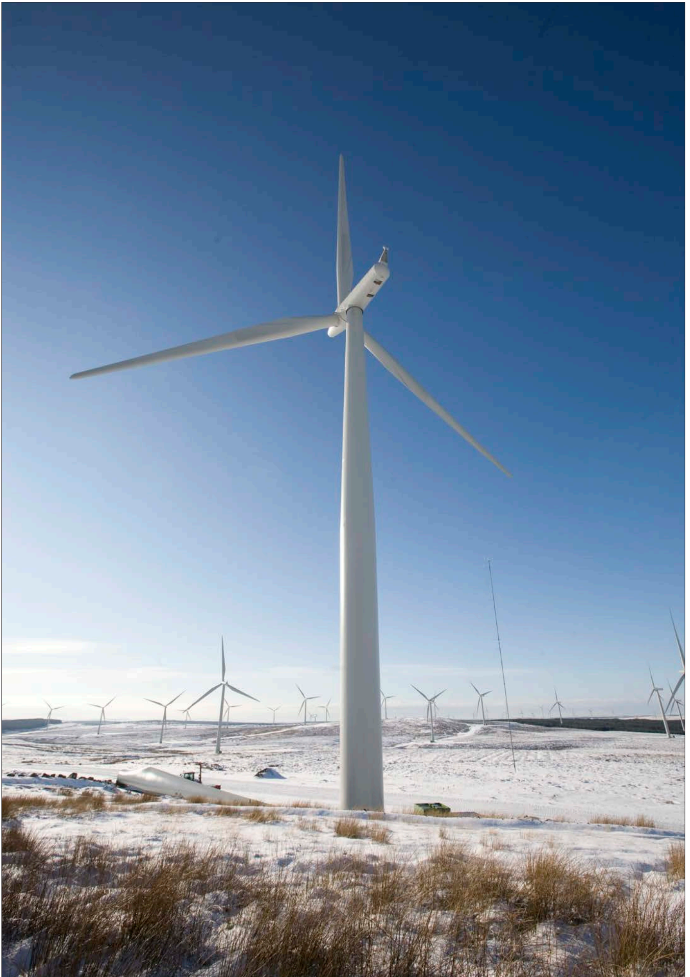
Above: Scottish Power's Whitelee windfarm – the largest in the UK
