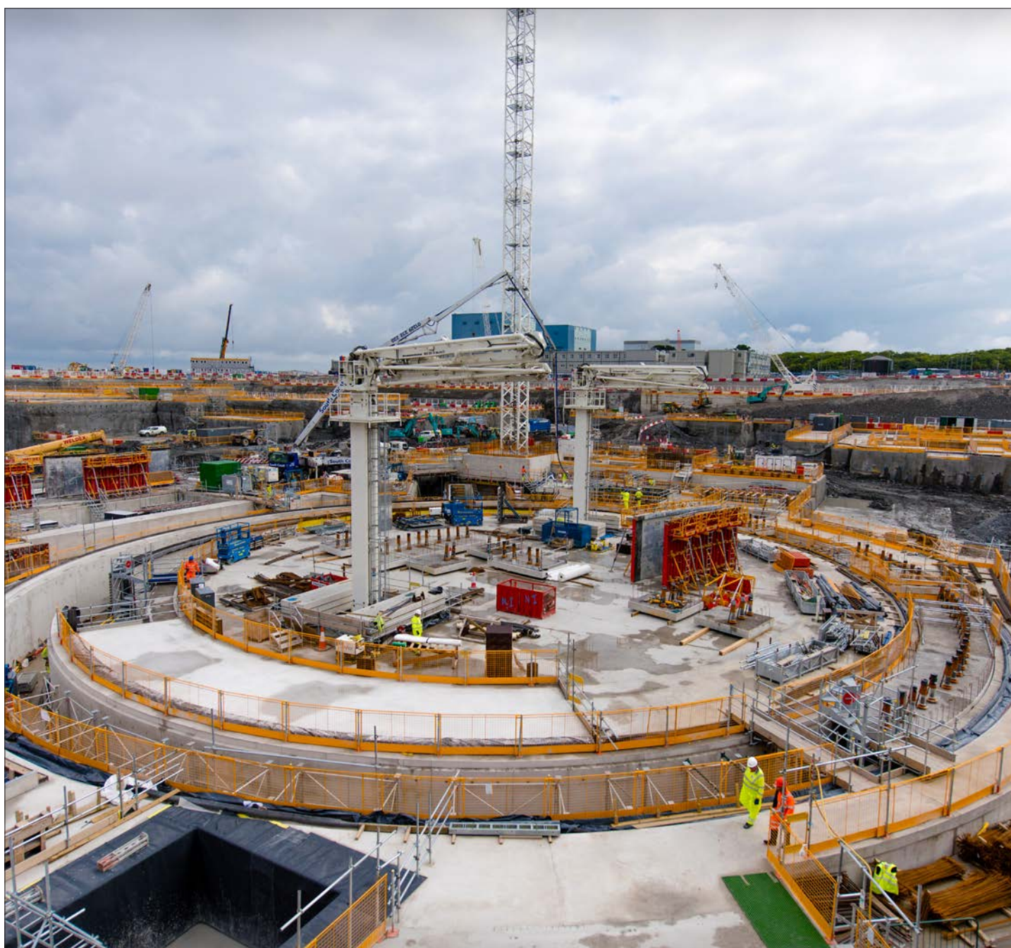
Above: Construction work at Hinkley Point C
